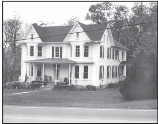
Clary's Mountain Historic District, Hedgesville Vicinity, Berkeley County
