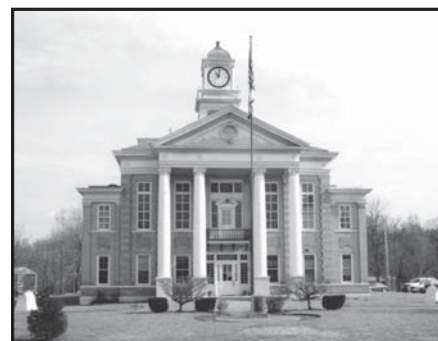
Wirt County Courthouse, Elizabeth
