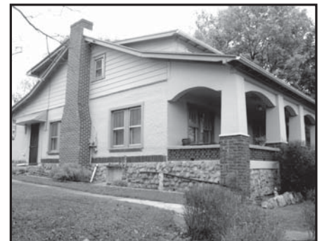
Benjamin H. Snyder House, Martinsburg Vicinity, Berkeley County
