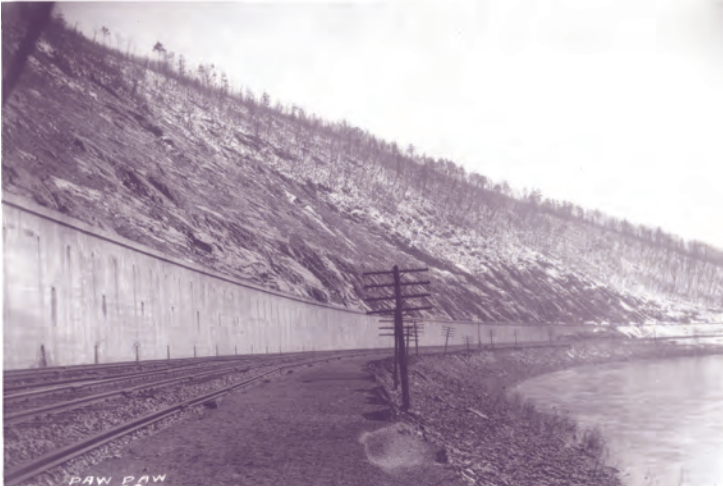
Just west of Graham Tunnel, the new tracks of the Magnolia Cutoff, separated by a massive concrete wall, were elevated above the old line. This separation earned the routes their respective designations of High Line and Low Line. Courtesy of B&O Railroad Historical Society.
