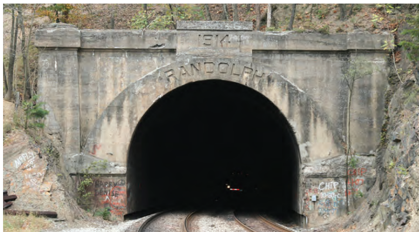
The name and completion date were incised into the portals of the tunnel.
