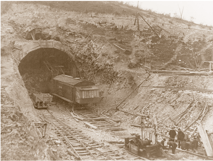
Steam shovels like this were used to open up and excavate the new tunnels associated with the Magnolia Cutoff. Courtesy of B&O Railroad Historical Society.
