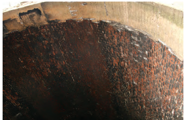
Tunnel interior showing brick lining.
